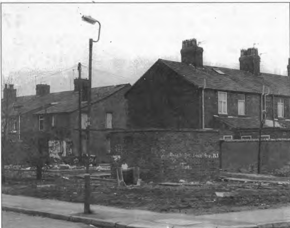
Before...! The usual view of this Manweb substation in the Tuebrook area of Liverpool.
