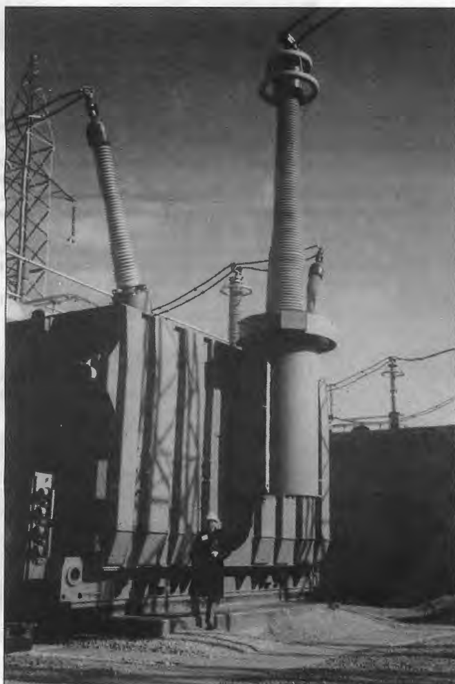
Even at 6ft 2in Arthur is dwarfed by one phase of the largest transformer in the world. The 3,000 MVA 765/345 kV transformer is at Marysville, Ohio.
