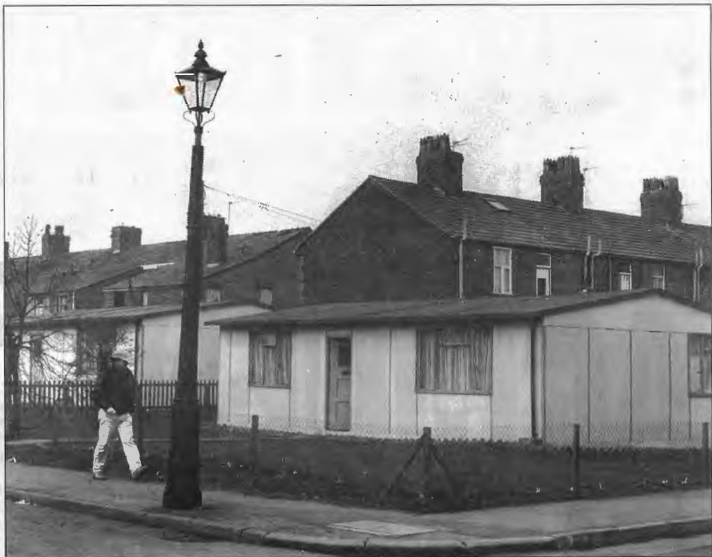
After...! The substation has been cleverly hidden under a typical 1940s prefab, to create an accurate 'post-war London' scene.
